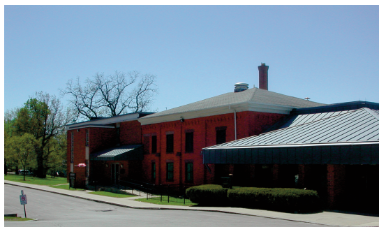
The Livingston County Jail will receive a new boiler system and energy efficient lighting
